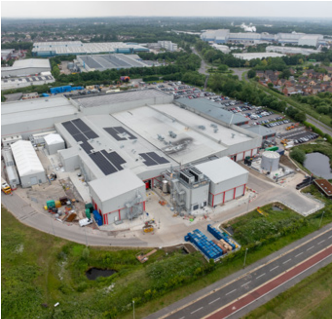
The Bradgate Bakery site including the new extension and solar panels
